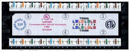
The 110 termination blocks are color coded for easy wiring identification.
